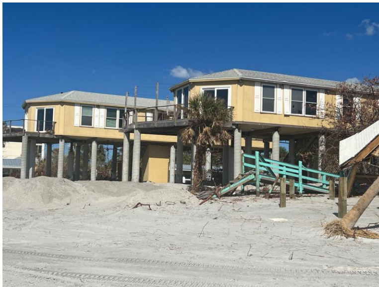
Figure 5: Elevated buildings, on the coast in Manasota Key, suffered minimal damage.
