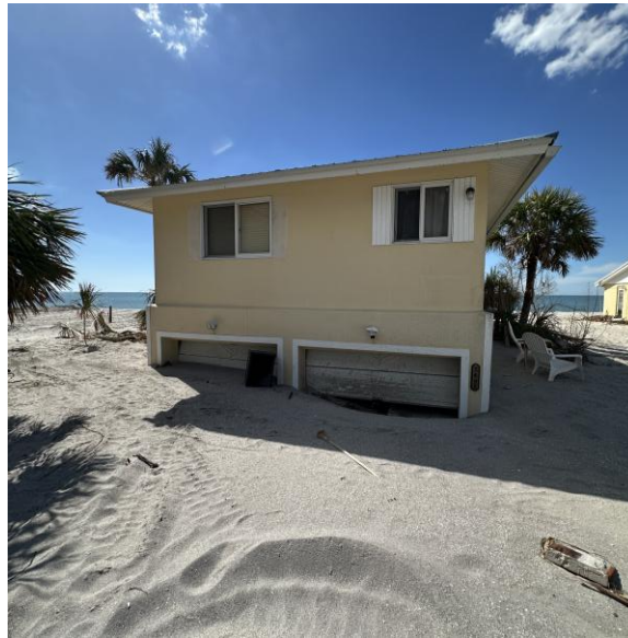
Figure 4: A coastal house that is covered in 3-4 ft of silt and mud in Manasota Key.
