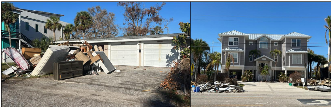
Figure 3: Widespread damage to interiors and content was found in most of the surveyed residential neighbourhoods
