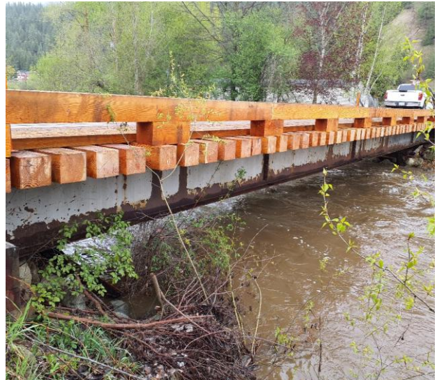
b) Typical low clearance farm bridge.
