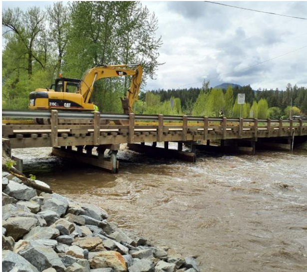
a) Multi-pier bridge with debris being removed
